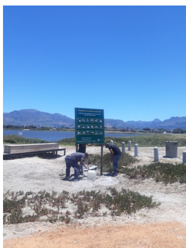
Left: Temporary icon signage erected on the Eastern shore, Princess Vlei.
